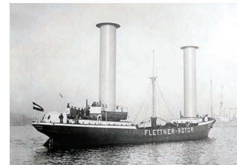
Figure 3.12 The Flettner rotor ship Baden-Baden , formerly the Buckau . Image courtesy of Wikimedia Commons
